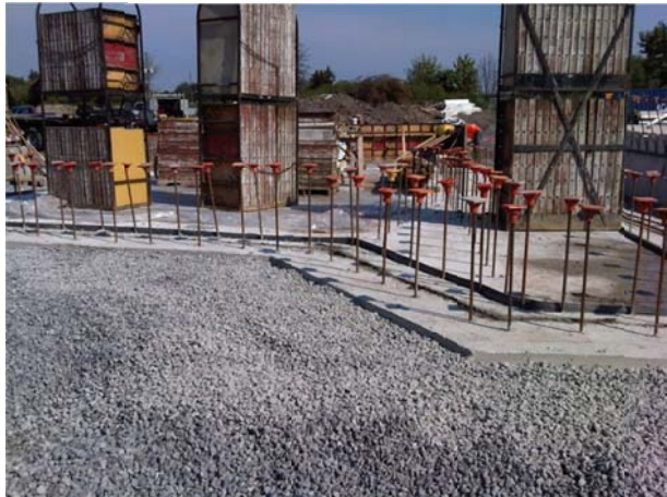
Leisure pool concrete formwork and pouring is ongoing
