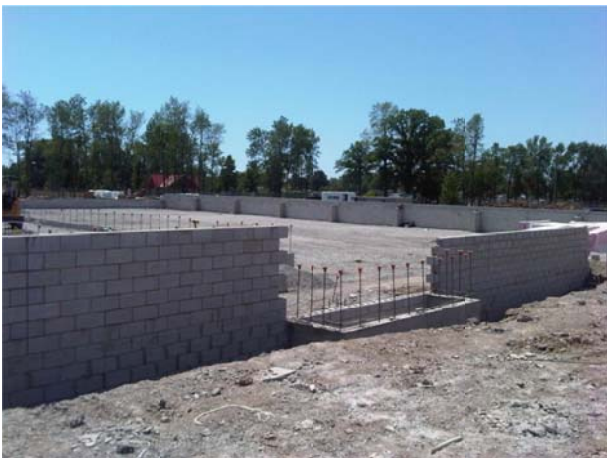
Arena 2 ready for steel
