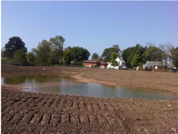
Storm water management pond ready for seed
