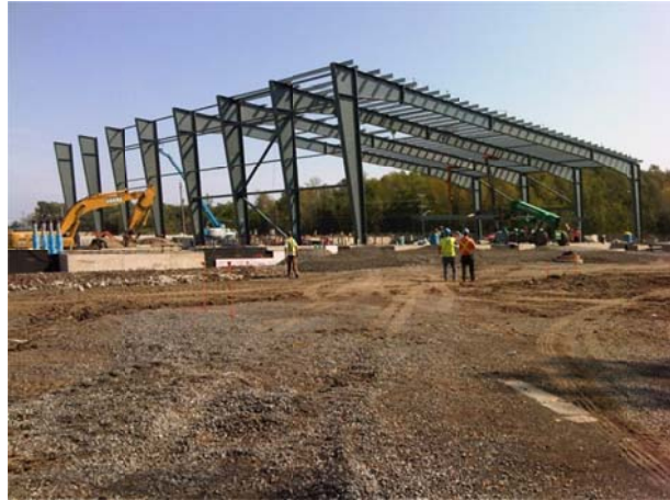
Arena 1 steel erection ongoing
